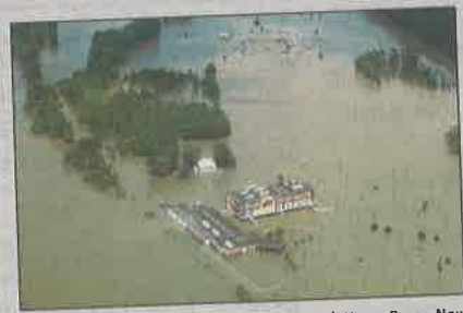
File photo | News-Press Now The 2011 flood surrounded former Terrible's Casino, now St. Jo Frontier Casino. A judge has ruled the Army Corps of Engineers were responsible for flooding and damage in four states.
